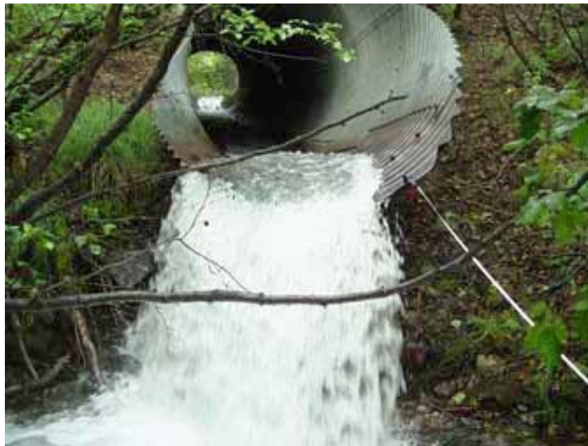
FIGURES 1 & 2. Excessive water drop and high velocity water flow impedes or blocks fish migration. © Jerilyn Walley/South Puget Sound Salmon Enhancement Group; Washington Department of Fish and Wildlife.
